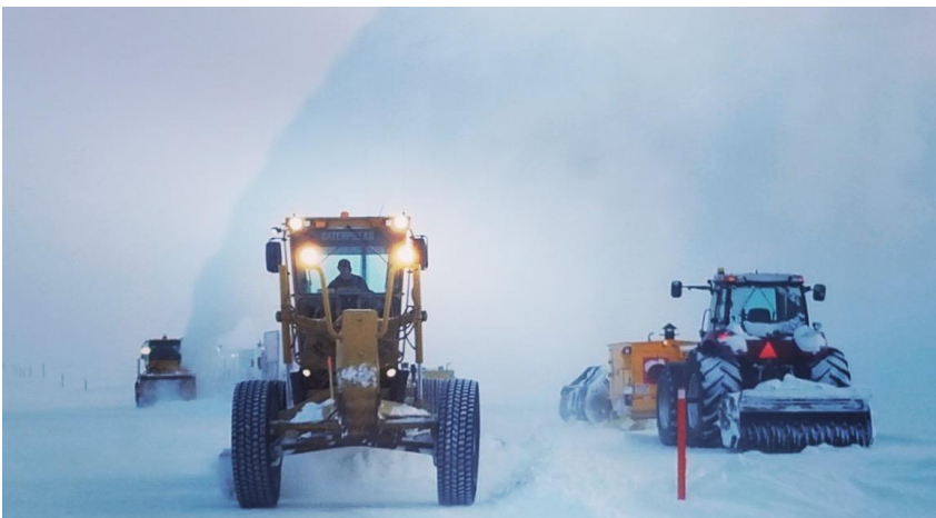
Figure 1 | Ice road construction.
