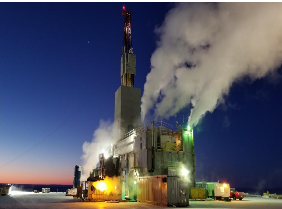
Figure 1 | Nordic Rig #3 on location, drilling ahead
