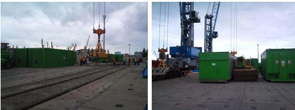
Figure 1 & 2 – unloading of equipment at the Port of Poti, Georgia
