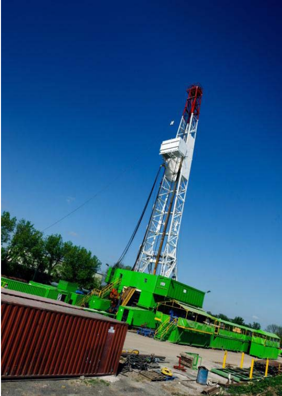
Figure 3 – Edeco Drilling Rig
