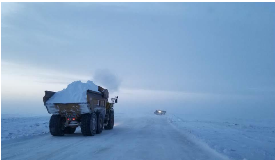
Figure 1. Ice road construction for Winx-1
