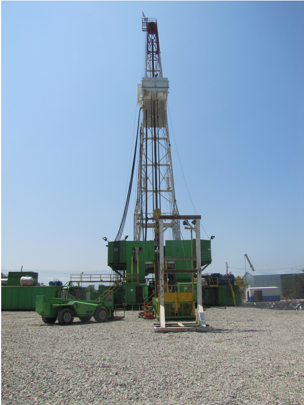
Drilling Rig on the Mukhiani Well site
