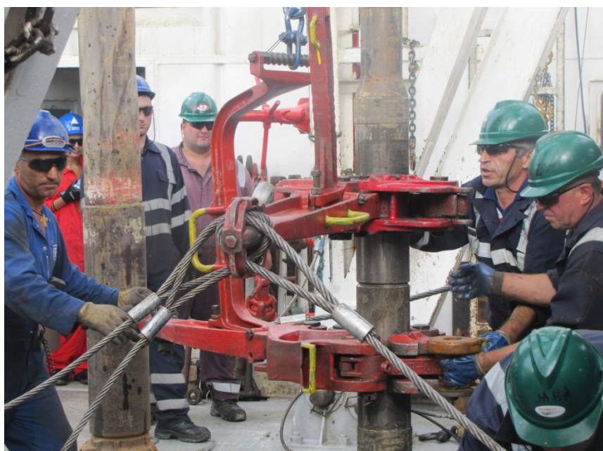
Figure 2 – Drilling operations – Mukhiani #1 Well
